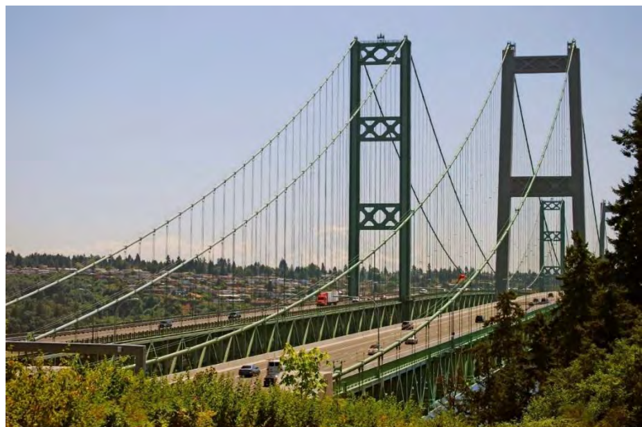
Tacoma Narrows Bridge
