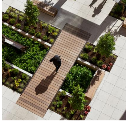
Bioretention facility in plaza / open space
