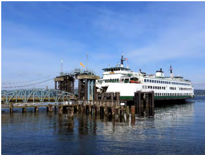
Mukilteo Ferry Dock
