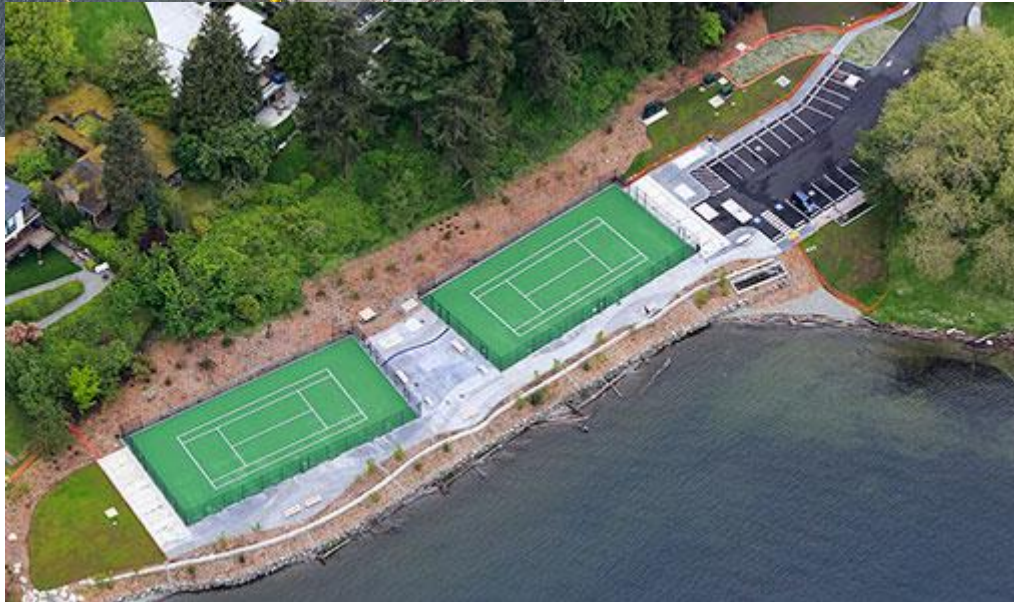
North Henderson Combined Sewer Overflow Reduction
