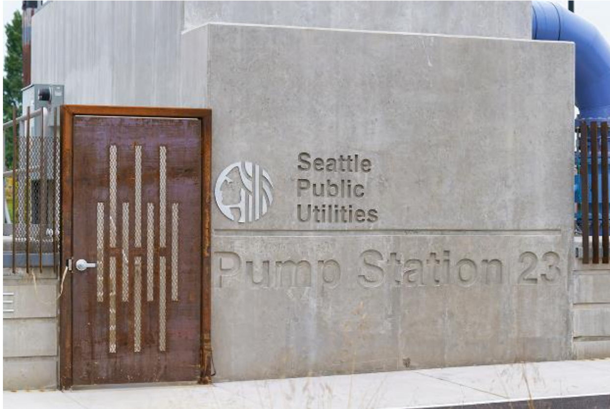
South Park Pump Station
