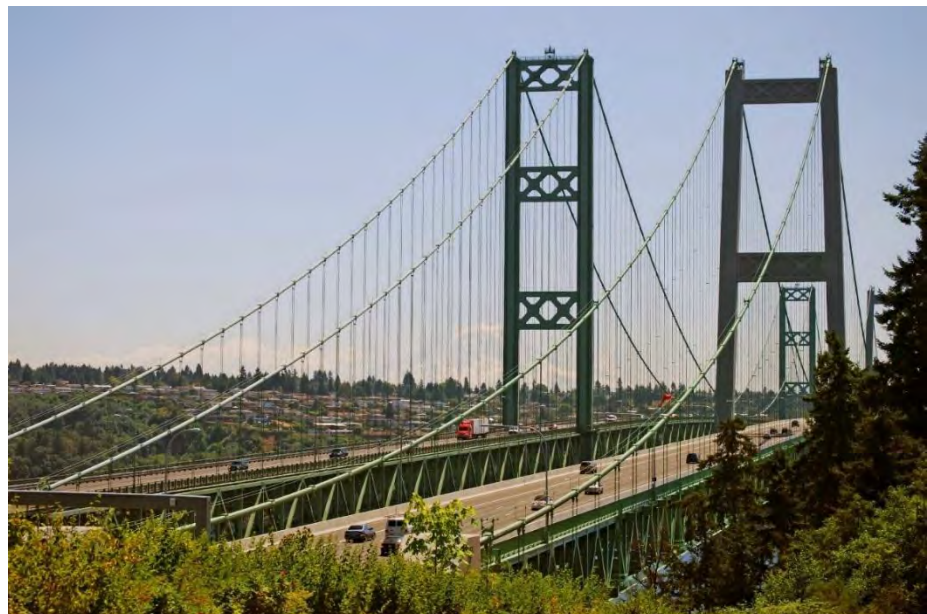
Tacoma Narrows Bridge
