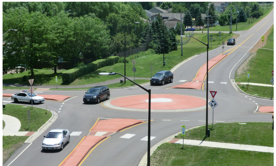
Example of a single-lane roundabout. Source: FHWA
