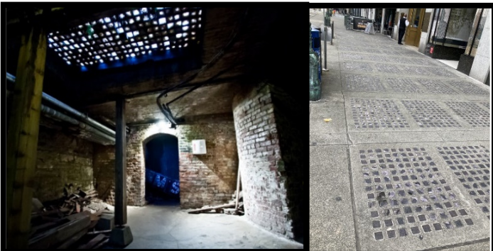
Throughout Pioneer Square, stained glass imbedded in the sidewalks provide light to the historic areaways below, and also enhance the unique character of the modern streetscape above.
