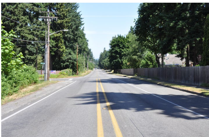
Figure H: Improvements Under Construction on Shaw Road
