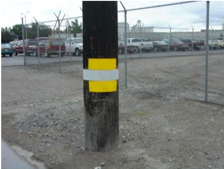
FIGURE 15. UTILITY POLE OBJECT MARKERS 18
