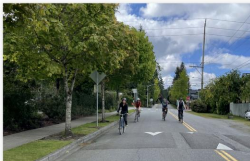
Road safety improvements using speed humps
