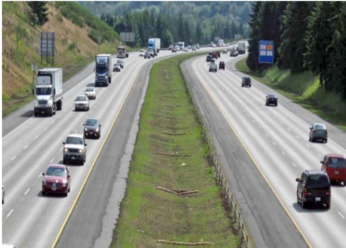
Compost Amended Vegetated Filter Strip
