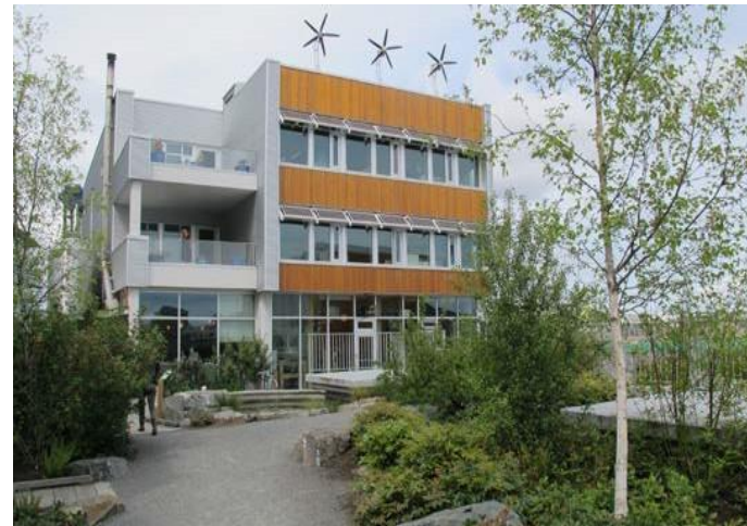
Safe street crossings and shared-use paths to add bike/ped circulation. Sustainable design opportunities, especially in the SW.
