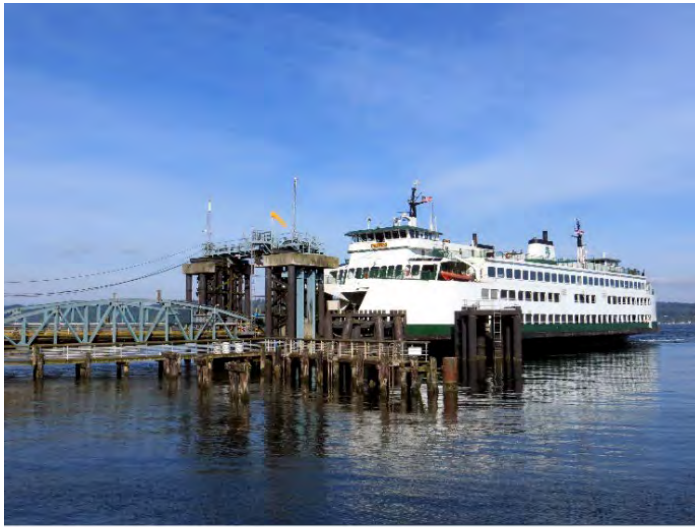
Mukilteo Ferry Dock
