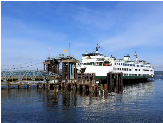
Mukilteo Ferry Dock
