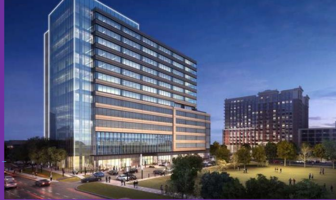
Facade with vertical and horizontal articulation; Integrated with streetscape and park.
