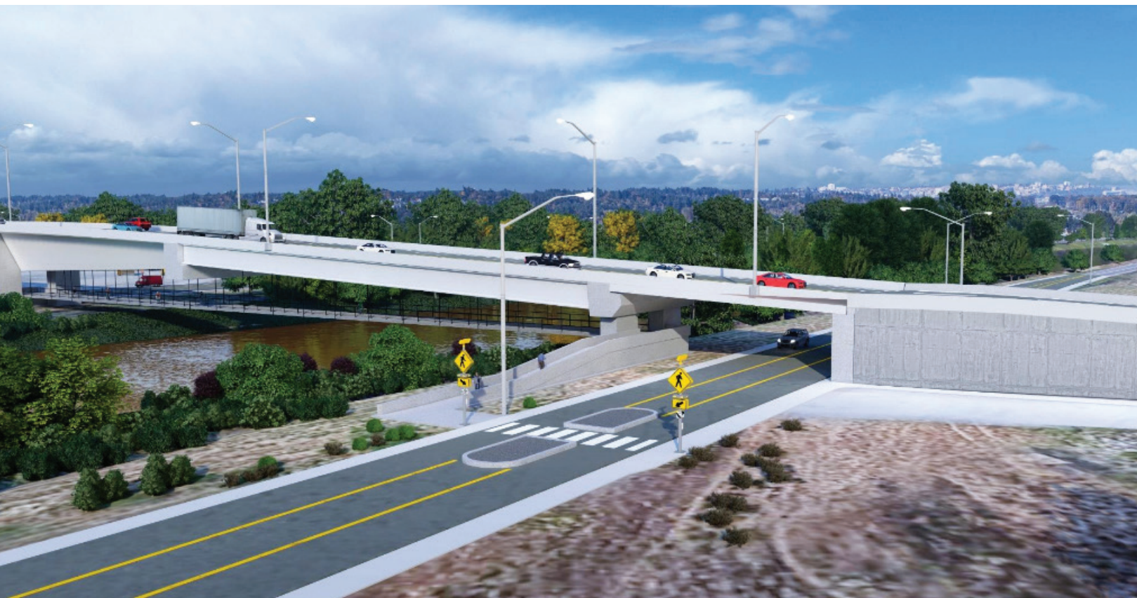
Pierce County received $4 million for the Canyon Road Freight Corridor Improvements project, which will include building a new bridge over the Puyallup River.
